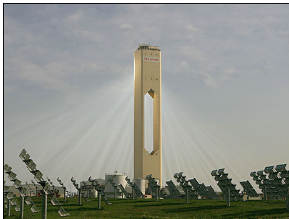
A field of more than 600 huge mirrors angled to reflect the sunlight of Andalusia onto a concrete tower. The heliostat mirrors track the progress of the sun, harvesting its power. The mirrors reflect and focus the sun's rays to the top of the tower where heat of 250C is absorbed and transmitted to a steam-driven generator. It is Europe's first commercially operated power station. Its operator, Solucar, claims that it generates 11 Megawatts of electricity. The energy it produces is enough to power up to 6,000 homes. Eventually it should produce enough power to supply the needs of Seville's 600,000-strong population.
