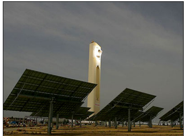
A field of more than 600 huge mirrors angled to reflect the sunlight of Andalusia onto a concrete tower. The heliostat mirrors track the progress of the sun, harvesting its power. The mirrors reflect and focus the sun's rays to the top of the tower where heat of 250C is absorbed and transmitted to a steam-driven generator. It is Europe's first commercially operated power station. Its operator, Solucar, claims that it generates 11 Megawatts of electricity. The energy it produces is enough to power up to 6,000 homes. Eventually it should produce enough power to supply the needs of Seville's 600,000-strong population.
